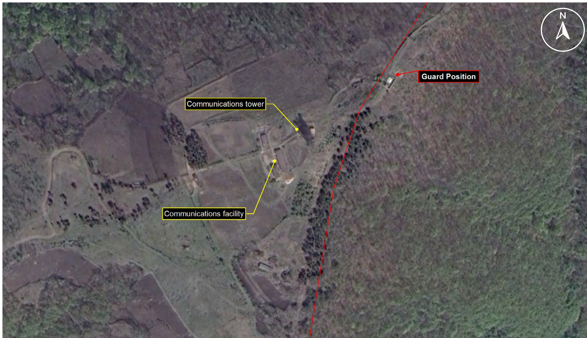
Area 21 - Communications Facility
