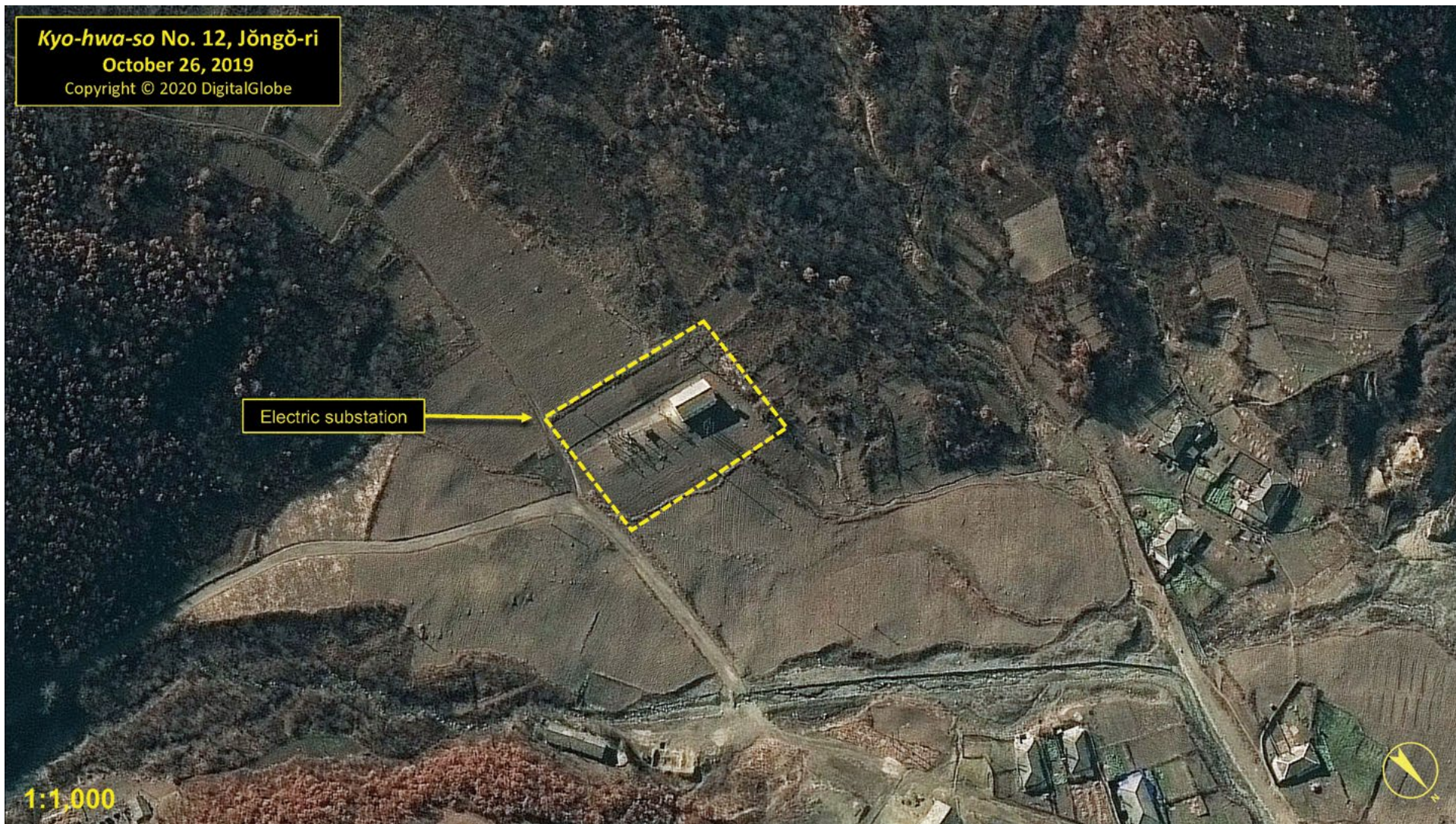
Electric substation (42.1998 N, 129.7546 E), October 26, 2019. (Copyright © 2020 by DigitalGlobe)
