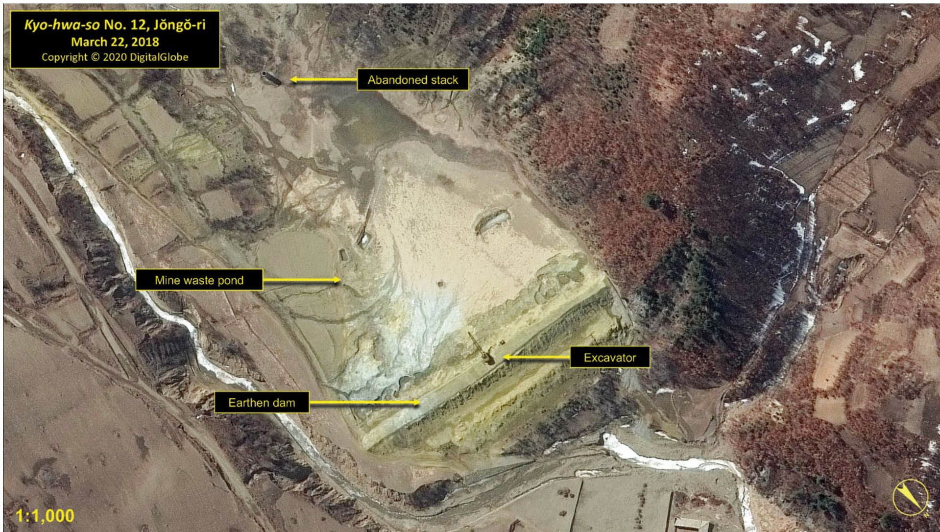
Copper mine waste pond (42.2058 N, 129.7528 E), March 22, 2018. (Copyright © 2020 by DigitalGlobe)
