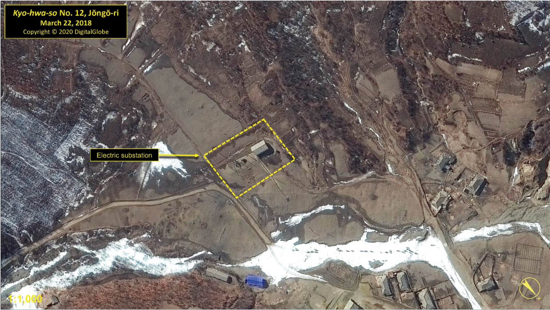
Electric substation (42.1998 N, 129.7546 E), March 22, 2018. (Copyright © 2020 by DigitalGlobe)
