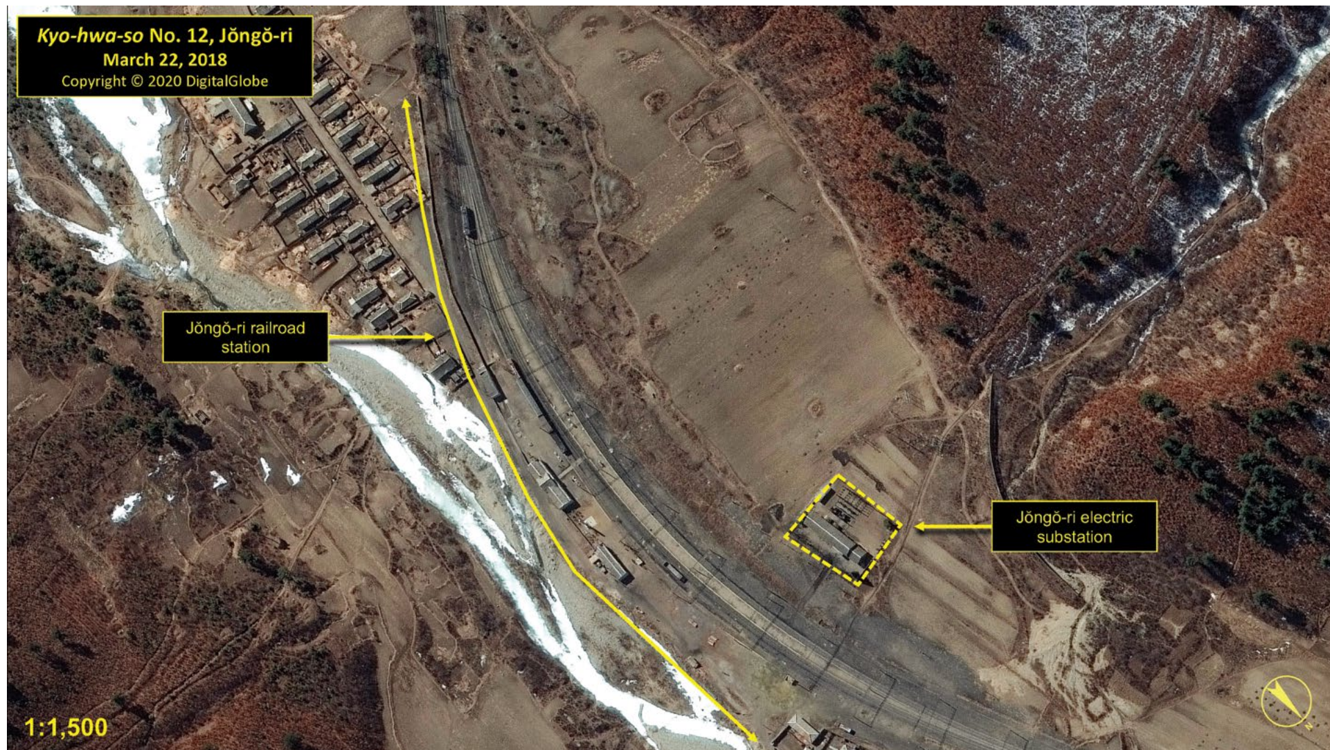
Jön'gö-ri railroad station and electric substation (42.2054 N, 129.7257 E), March 22, 2018. (Copyright © 2020 by DigitalGlobe)
