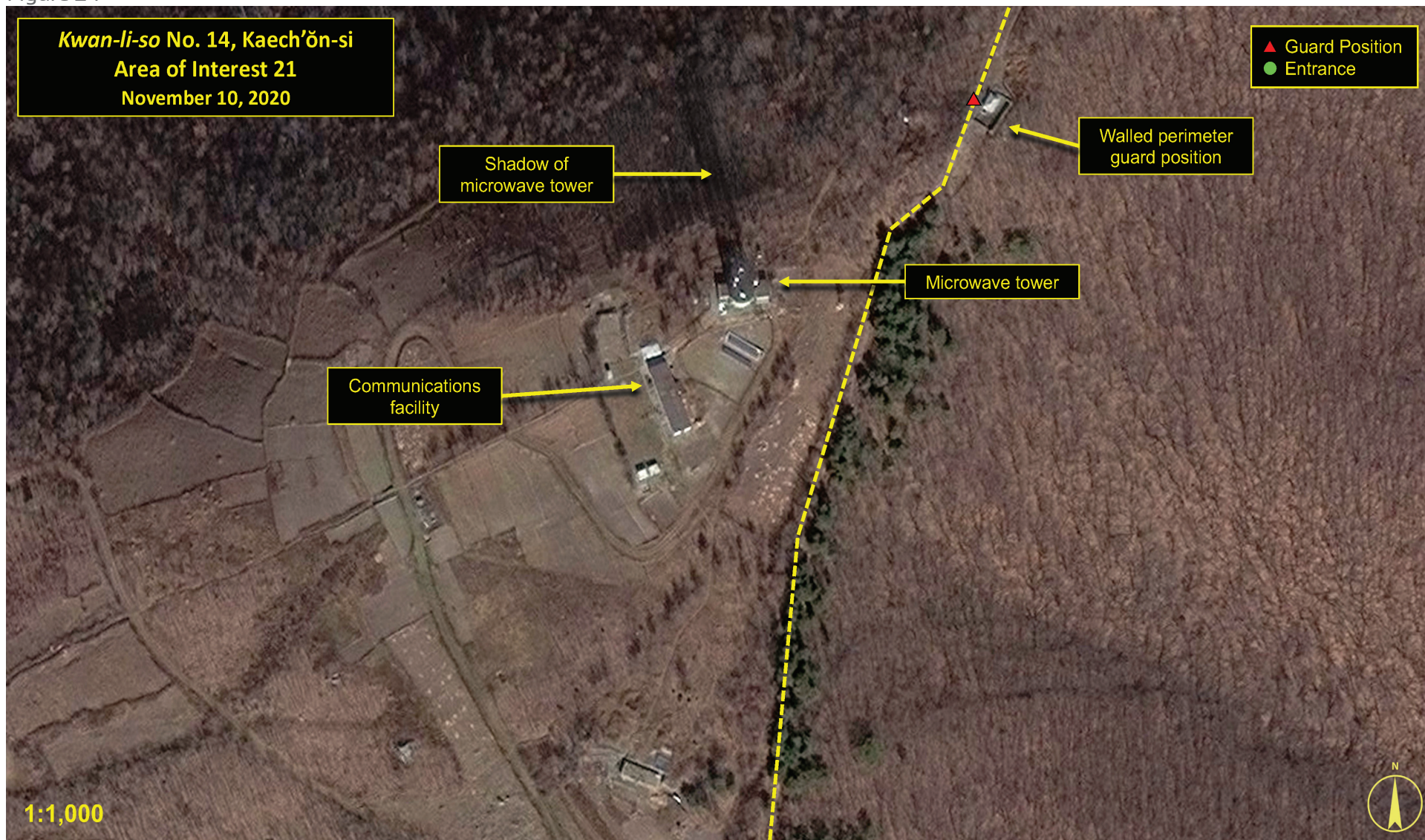
Area 21, Microwave Communications Facility
