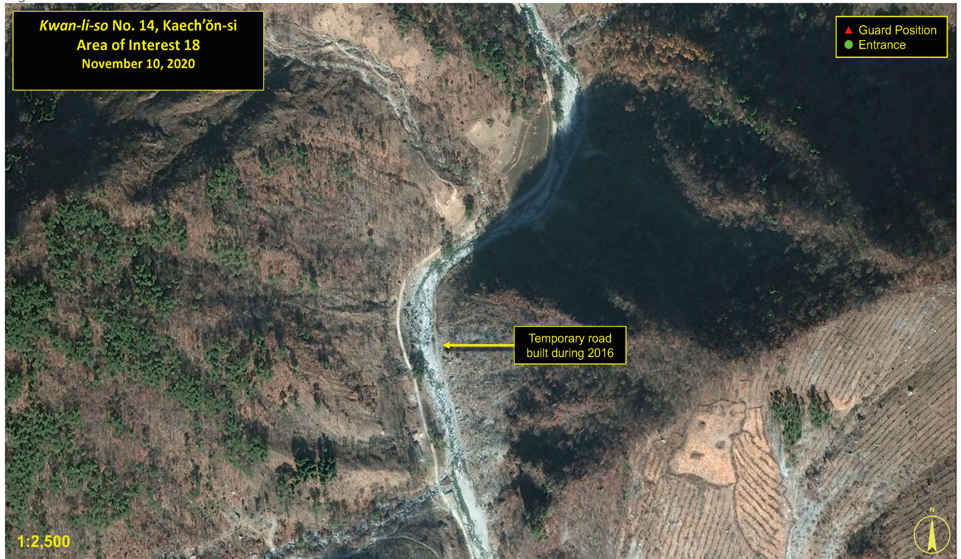
Area 18, Road Construction Completed
