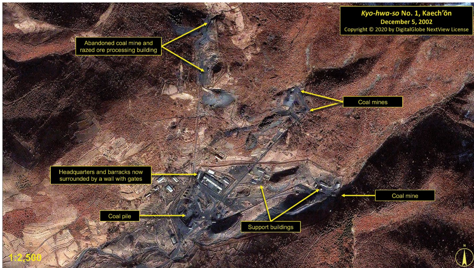
A view of the mining activity northeast of Kyo-hwa-so No. 1 showing that while the area is still active, the ore processing building has been razed and several mines appear to be abandoned. Additionally, the headquarters and barracks buildings have been enclosed by a wall with gates.
