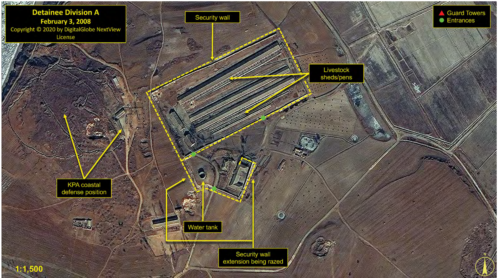
Figure 71: Reconfiguration of the livestock sheds/pens and portions of the security wall extension to the south and around the small building being razed, February 3, 2008. (Copyright © 2020 by DigitalGlobe, NextView License)
