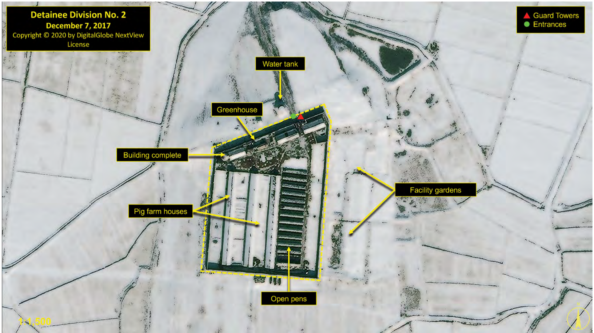
Figure 30: The construction of the fourth building inside Detainee Division No. 2 is complete, December 7, 2017 (Copyright © 2020 by DigitalGlobe, NextView License)
