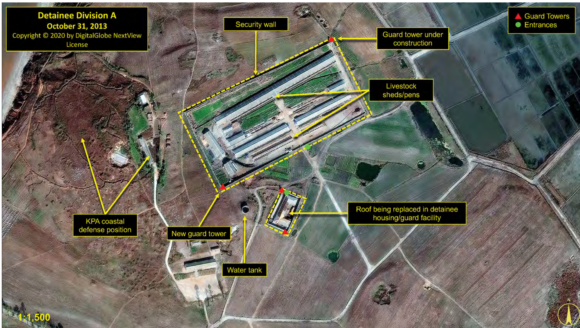
Figure 73: New guard towers visible on the security wall of Unidentified Detainee Division A, October 31, 2013. (Copyright © 2020 by DigitalGlobe, NextView License)
