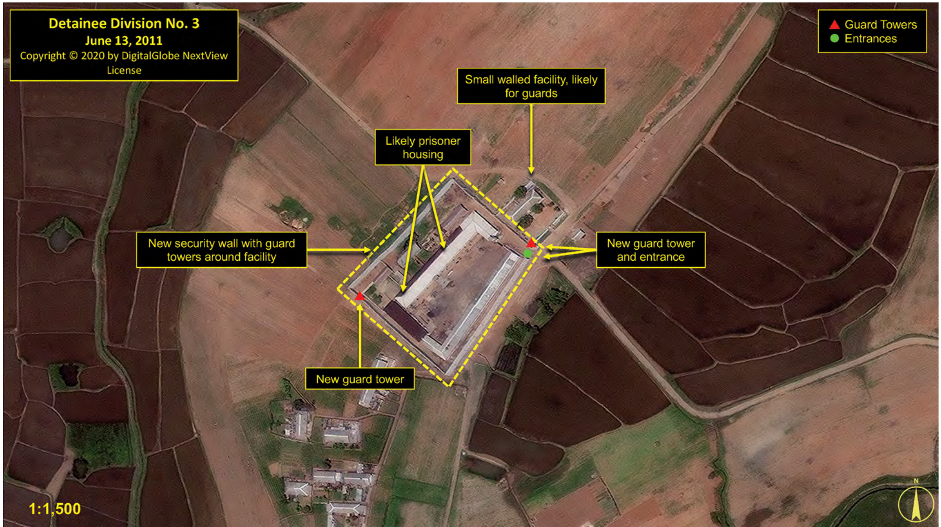
Figure 34: Detainee Division No. 3 on June 13, 2011. Several buildings have been razed, a new security wall has been erected around the entire detainee division and two guard towers added. (Copyright © 2020 by DigitalGlobe, NextView License)
