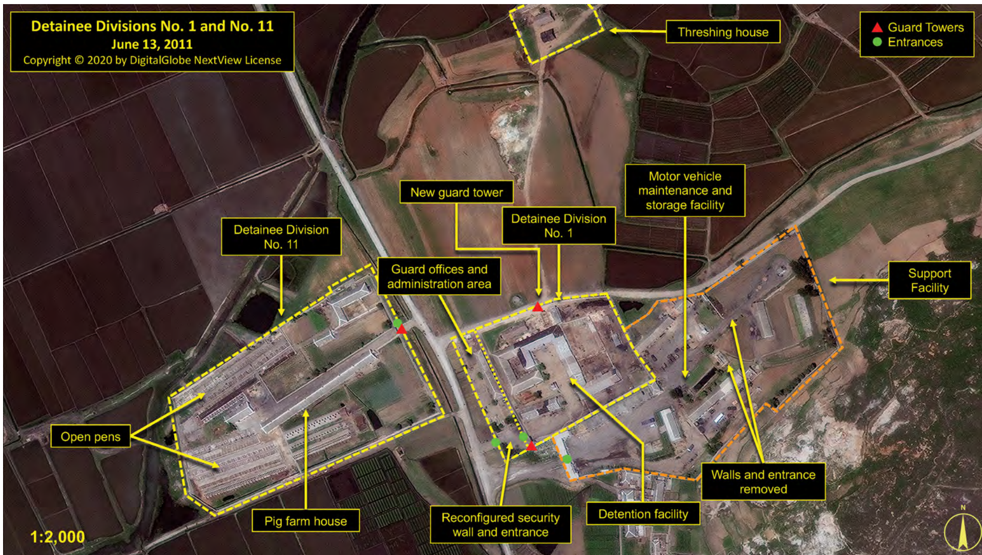
Figure 20: The reconfigured guard/administrative area and entrance, new guard tower on north wall and minor changes visible in the support area, June 13, 2011 (Copyright © 2020 by DigitalGlobe, NextView License)
