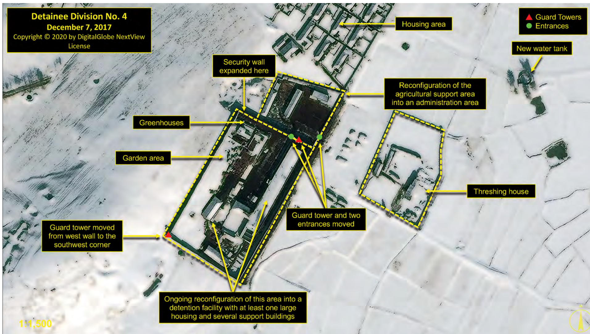
Figure 44: Significant changes to the administration and detention areas of Detainee Division No. 4 are seen in this December 7, 2017 image (Copyright © 2020 by DigitalGlobe, NextView License)
