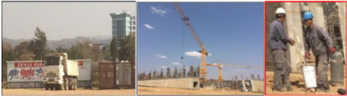
Figure 23 Construction at Suider Hof military base
